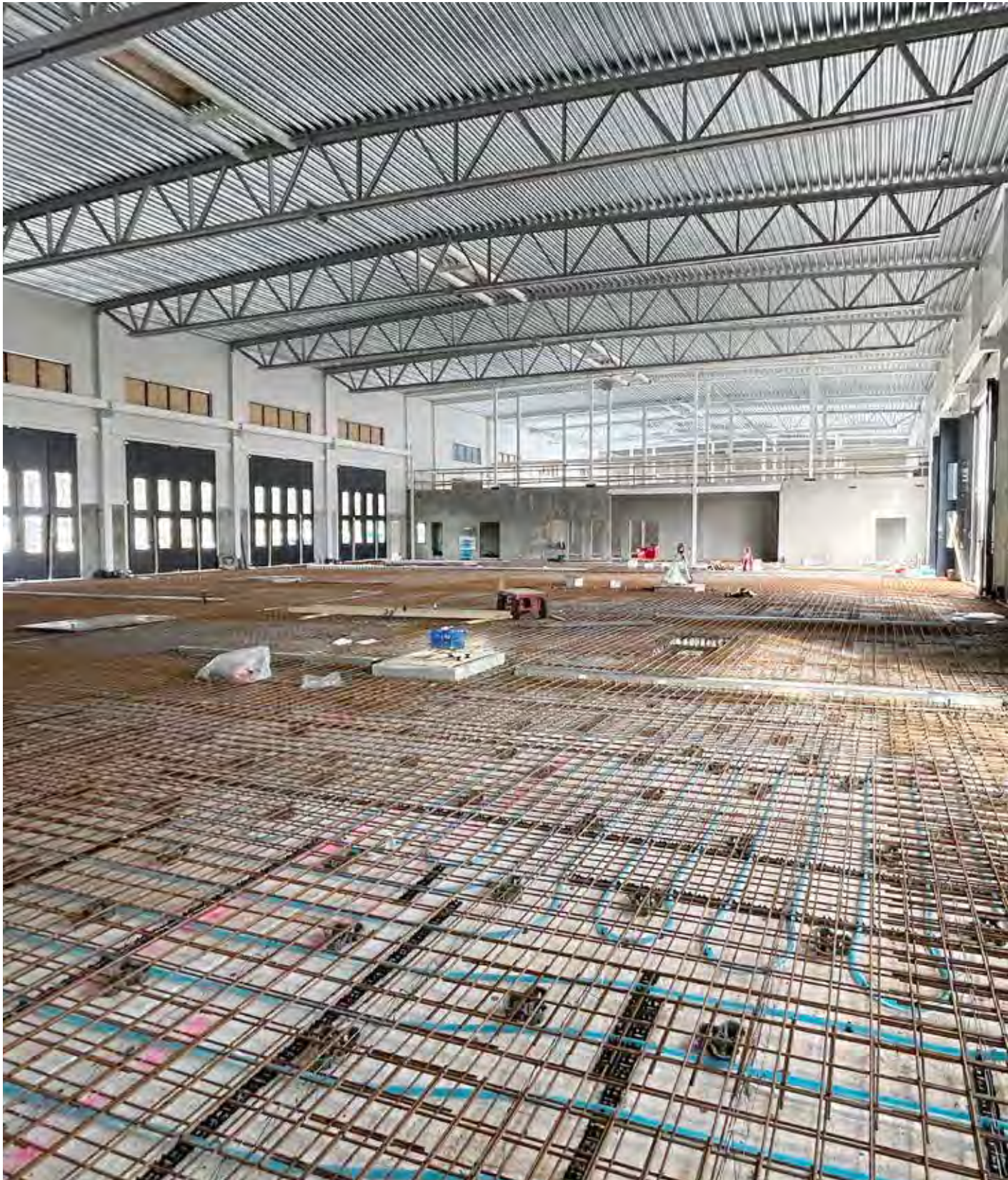
By the end of 2025, the construction of a new workshop for heavy vehicles for Berners in Östersund is expected to be completed. The total area amounts to 4,780 square meters.
