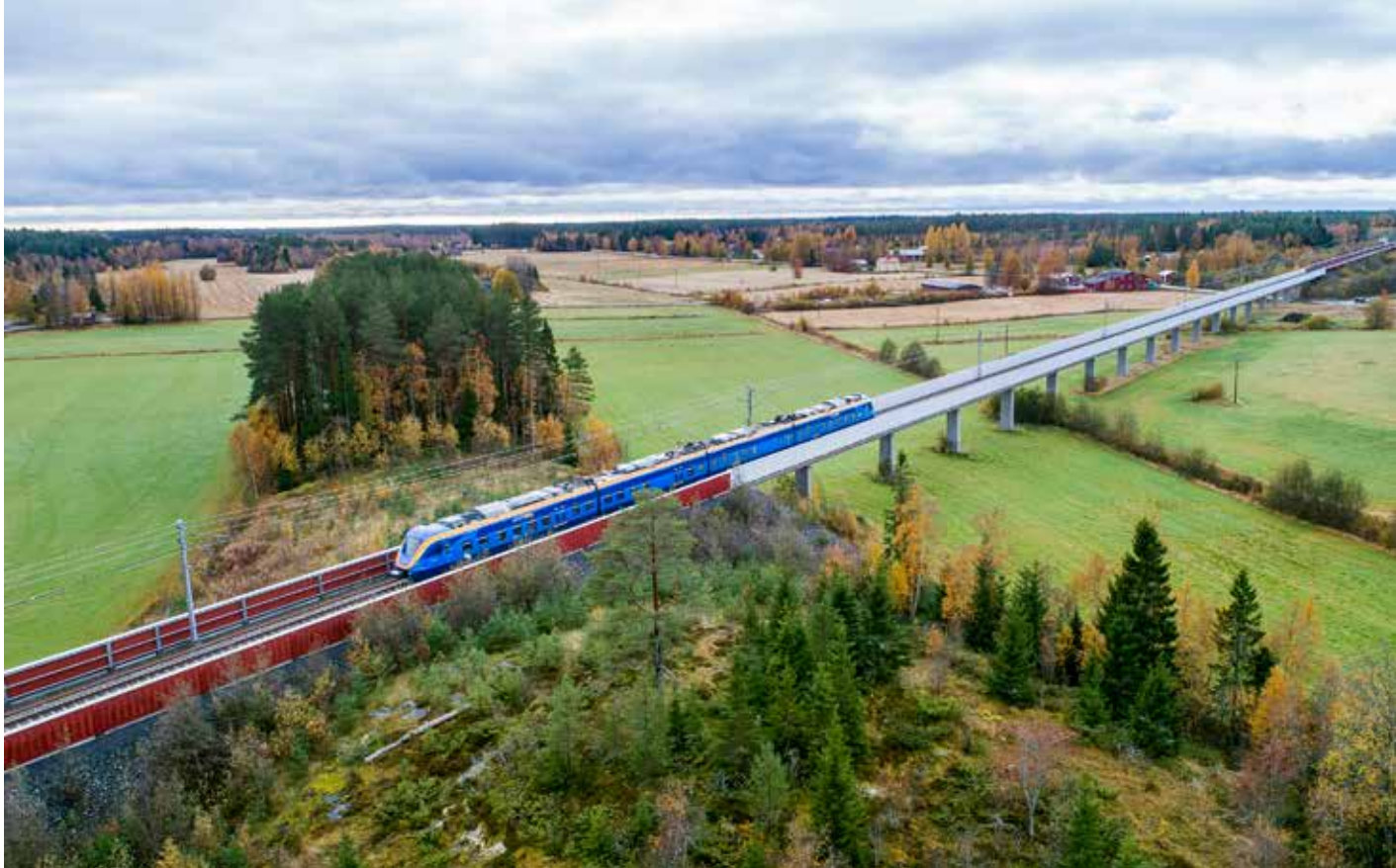
Major investments are planned in infrastructure in northern Sweden, including the North Bothnia Line, where BSEK 30 will be invested in railways.
